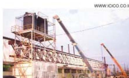
A 60-metre span lattice girder being erected for Automotive Axles Ltd in Mysore.
